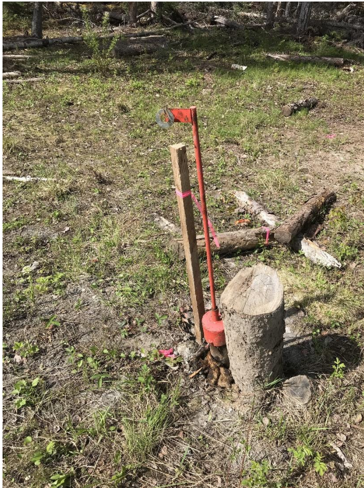
Figure 9-6: Drill hole location marked by metal flag
